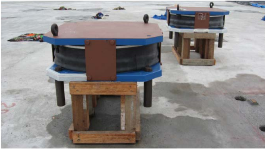
Picture C: Example Triple Pendulum bearings with 4 bottom shear-lugs connected.
