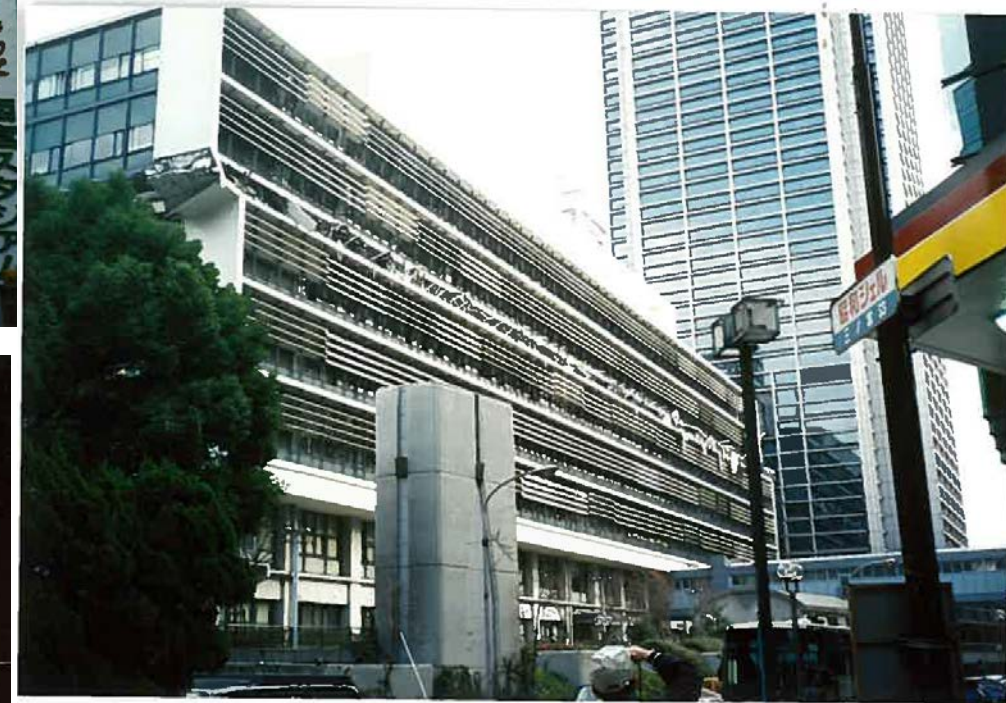
Kobe City Hall building
