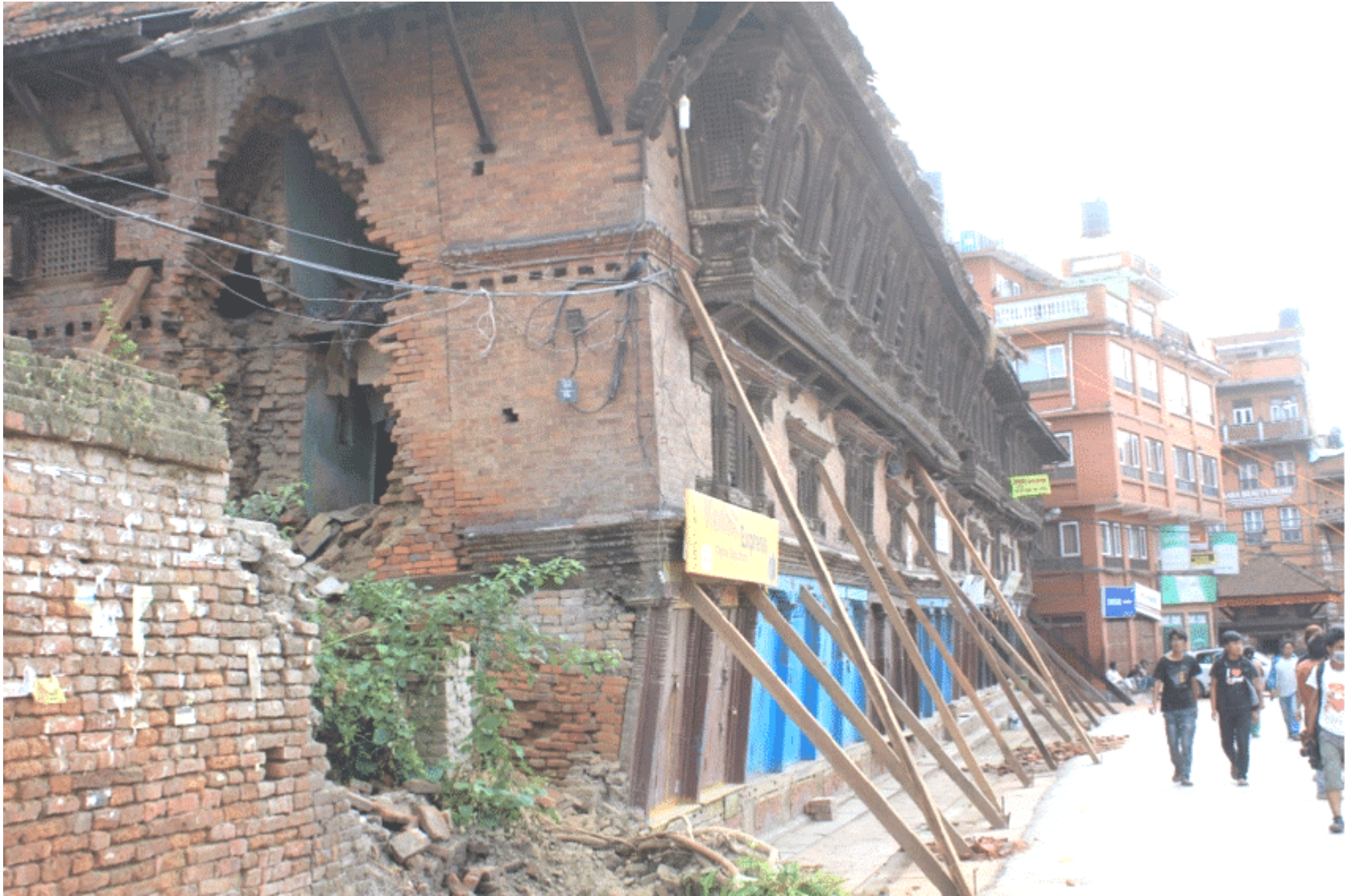
Collapsed unreinforced masonry building in Bhaktapur, Nepal following the Gorkha earthquake. Source: Ben Mason, 2015
