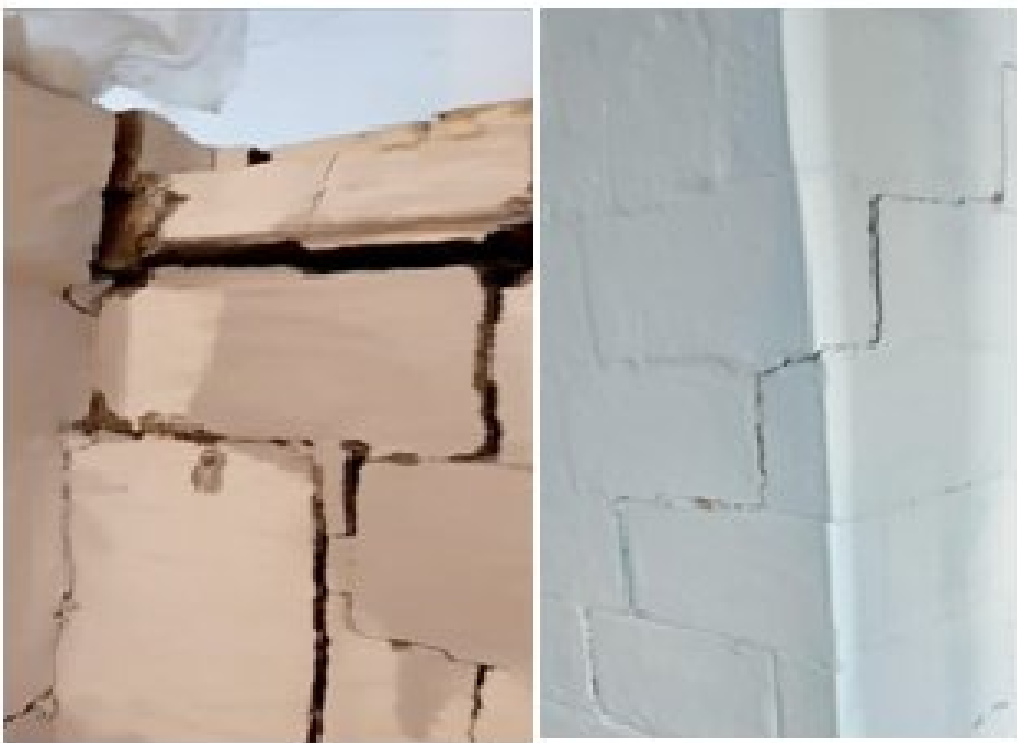
Figure 3. Cracking observed in the wall-mounted stove of a resident's home in Kosh-Agach village
